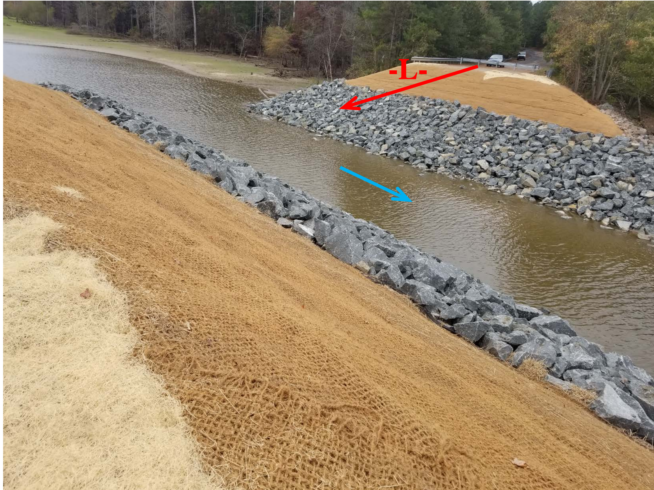
Looking West towards End Bent 1
